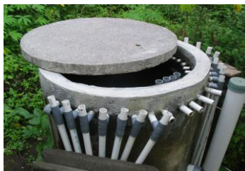
Gambar 12. Instalasi Distribusi Pengairan Tanaman Salak Pondoh
